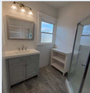
2nd floor bathroom: AFTER
