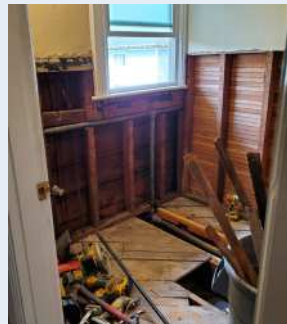
2nd floor bathroom: BEFORE
